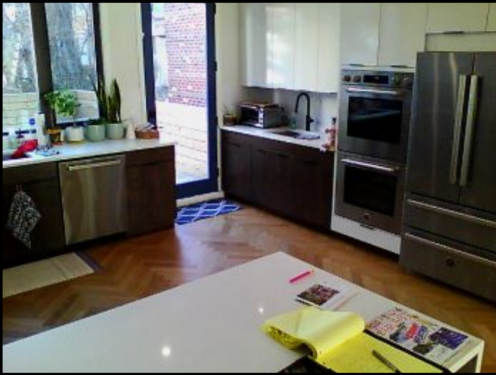
Severe draft entry point.
