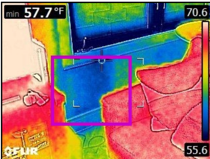
Infrared imaging of draft entry point.
