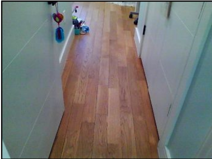
Floor board separation point. No indication of water entry within the area. Separation caused by improper installation.
