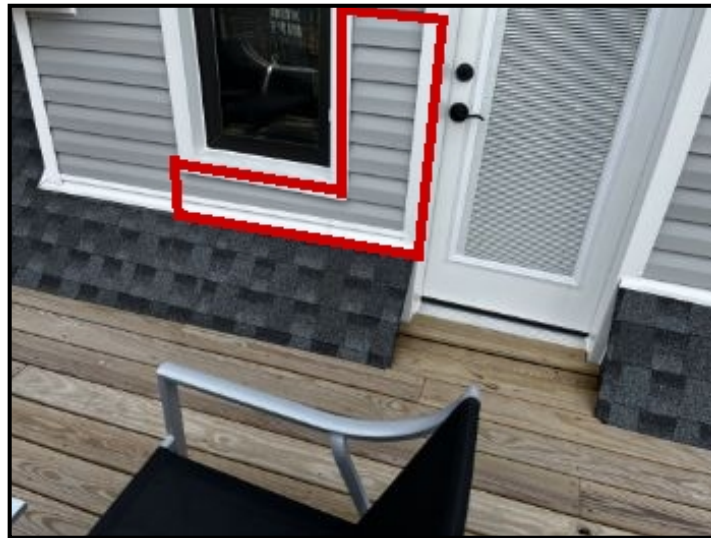
Repair Point: Remove siding from area. Waterproof area accordingly.
