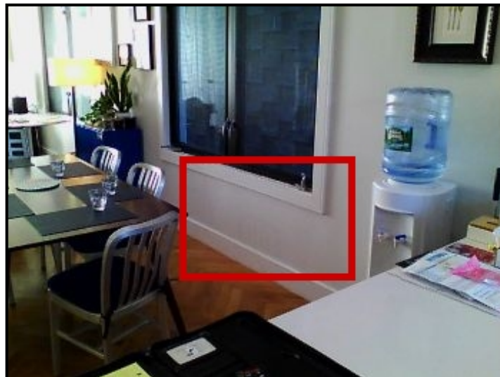
Repair Point: Excavate drywall. Install proper insulation.
