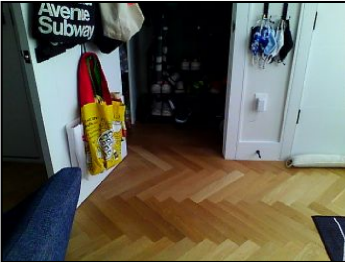
Severe draft entry point.
