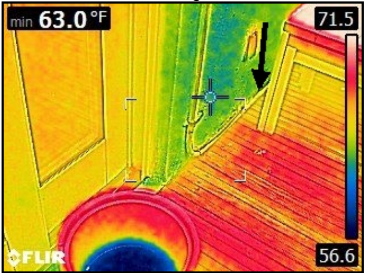
Infrared imaging of water entering through rear facade connection point to the deck system and cascading down into the wall/ceiling area below.
