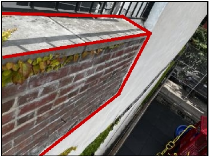
Repair Point: Waterproof parapet wall brick. Install aluminum flashing cap over parapet coping stone. Seal outer brick.
