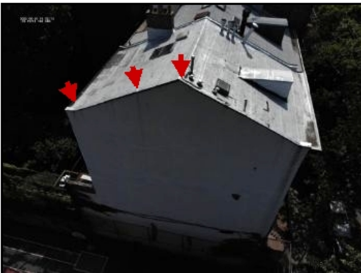
Repair Point: Inspect roof membrane system for continued viability. Install aluminum flashing cap over roof parapet wall.
