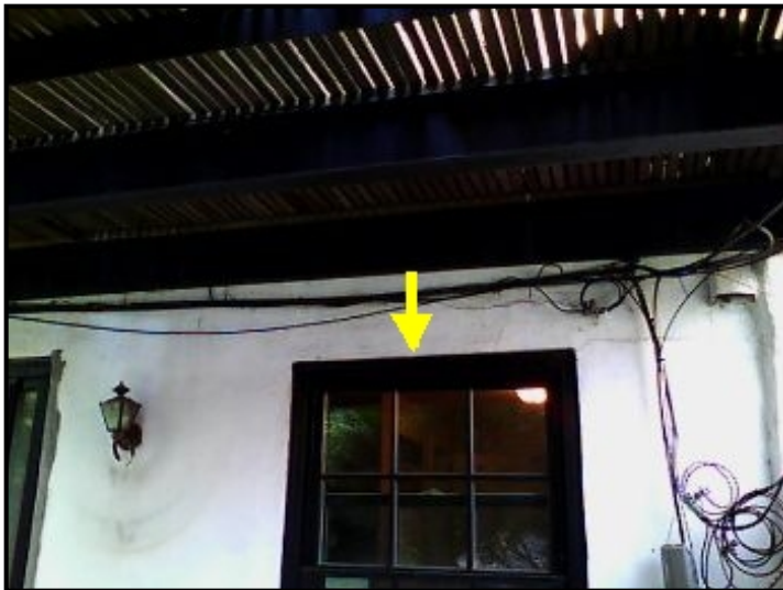
Water cascading down through rear facade and backflowing into the internal wall/ceiling area.
