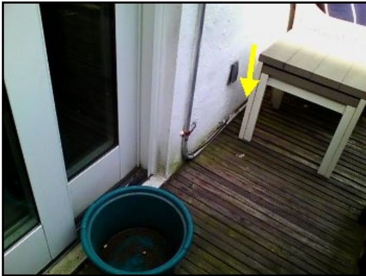
Water entering through rear facade connection point to the deck system and cascading down into the wall/ceiling area below.
