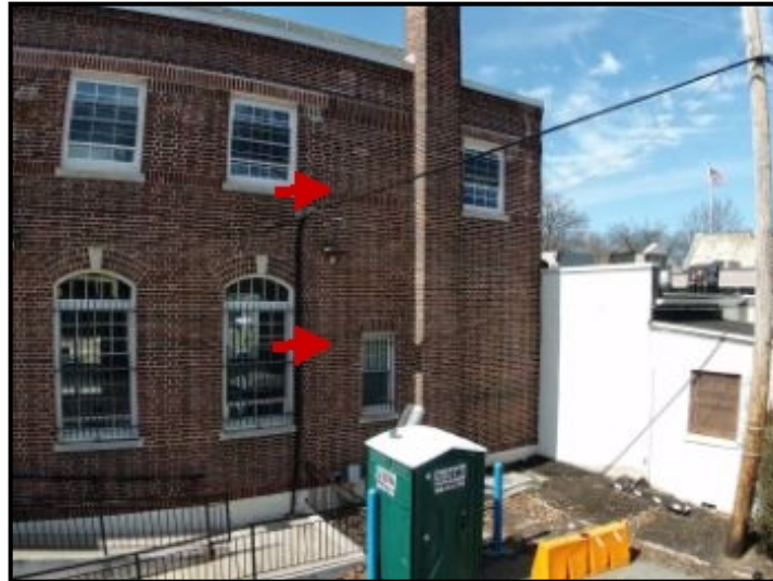
Repair Point: Seal brick facade with Silane Siloxane sx5000.
