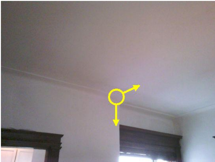
Water entry into wall area due to a combination of condensate buildup from the boiler exhaust discharge as well as water entry through the chimney walls and connecting parapets, cascading down and depositing into the wall areas below.
