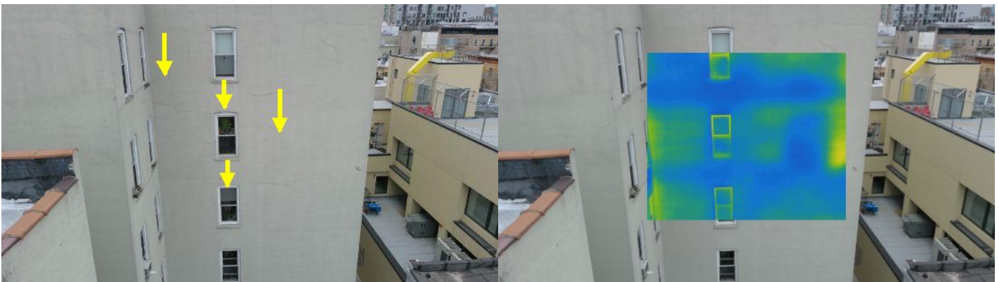
Water entering through the window sills and parapet wall coping stone, cascading down and depositing into the wall / window areas below.
