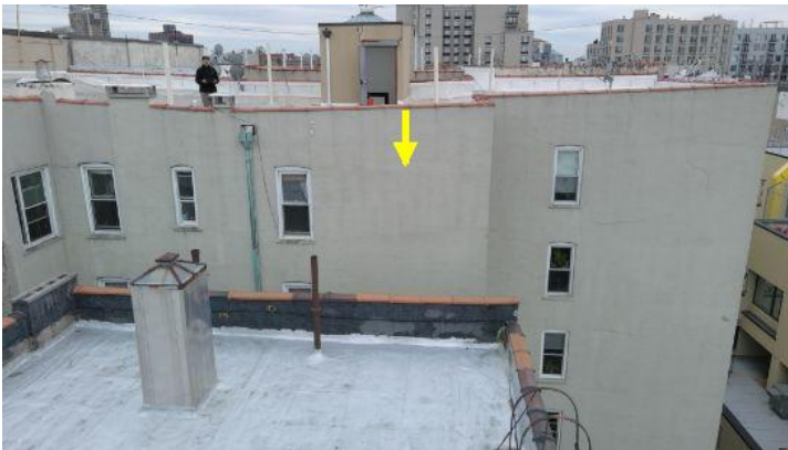
Water entering through side facade and parapet wall coping stone, cascading down and depositing into the wall areas below.
