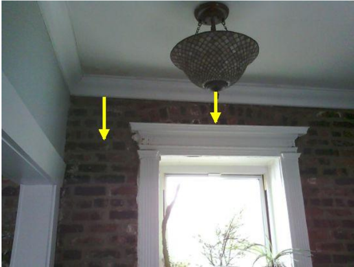
Water entry into wall / window frame area.
