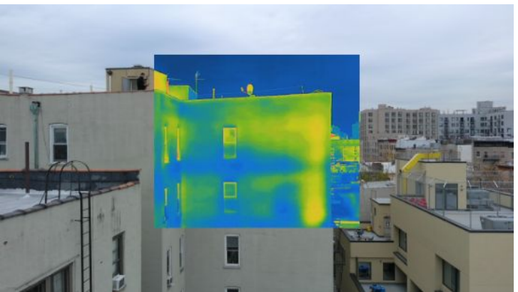
Infrared imaging of water entering through parapet wall coping stones and cascading down into the wall / window frame areas below.
