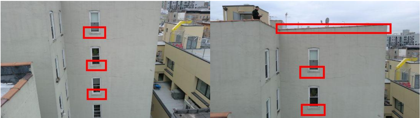
Repair Point: Waterproof window sills. Remove coping stone. Waterproof parapet wall.
