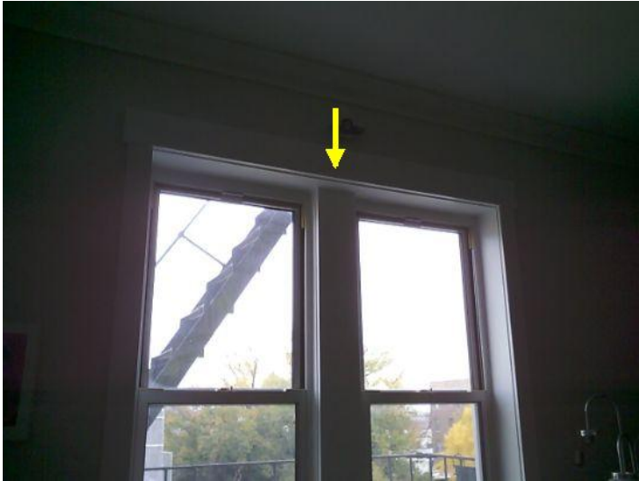
Water entry into wall / window frame area.
