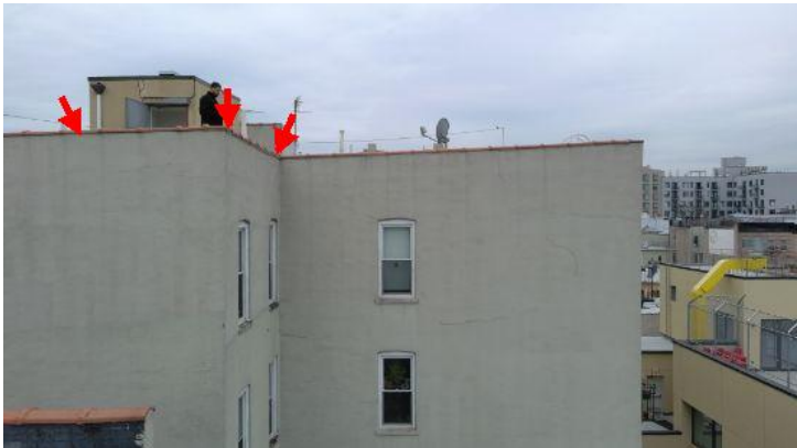
Repair Point: Remove coping stones. Waterproof parapet wall.
