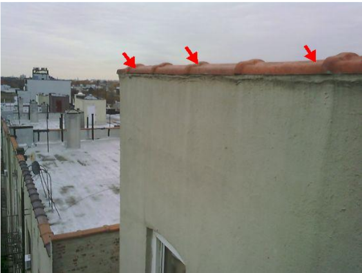
Repair Point: Remove coping stones. Waterproof parapet wall.
