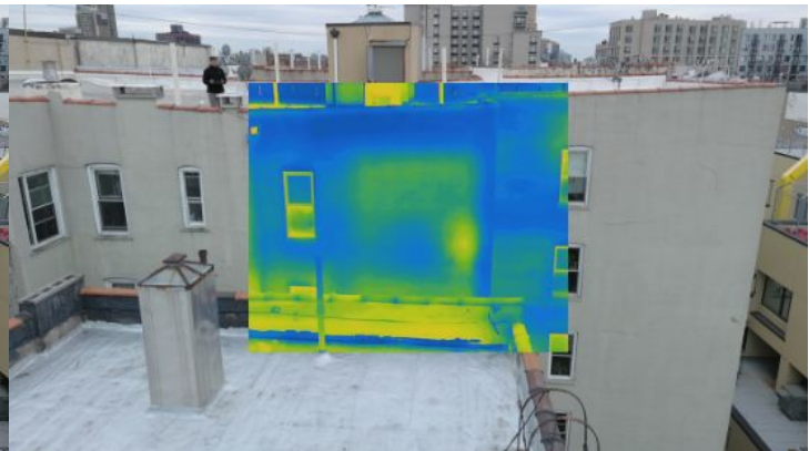
Infrared imaging of water entering through side facade and parapet wall coping stone, cascading down and depositing into the wall areas below.
