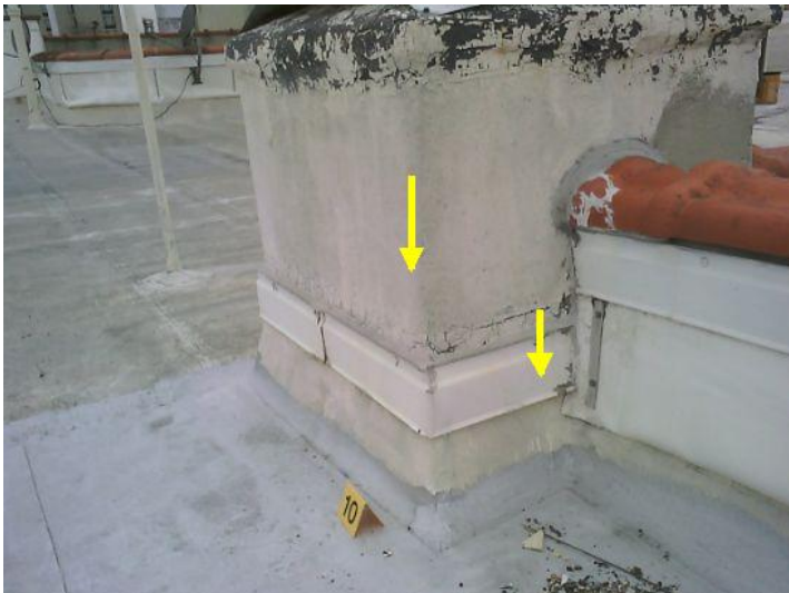
Water entering through the chimney structure as well as connecting parapet walls, cascading down and depositing into the wall areas below.
