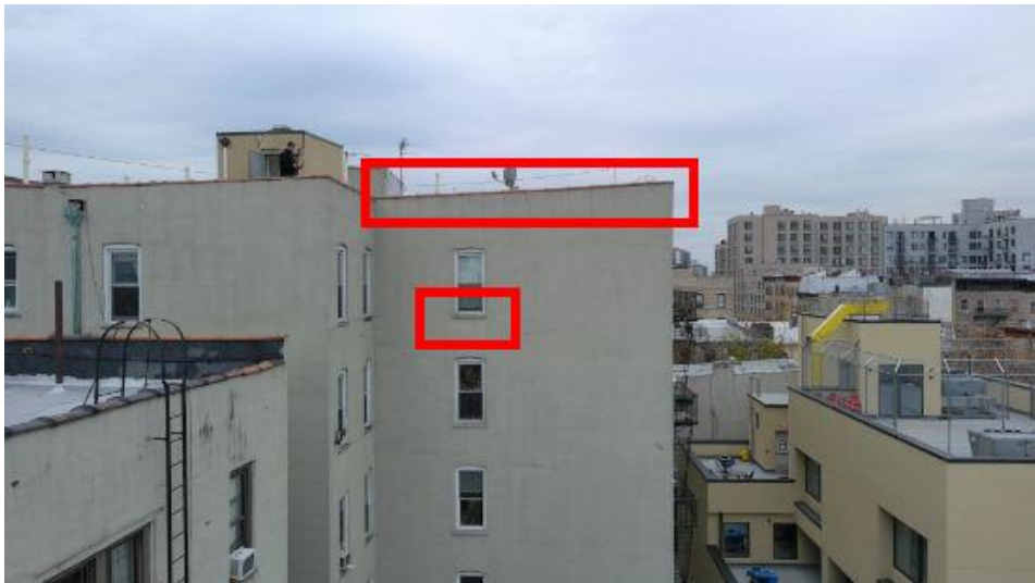
Repair Point: Remove parapet wall coping stones. Waterproof parapet wall.
