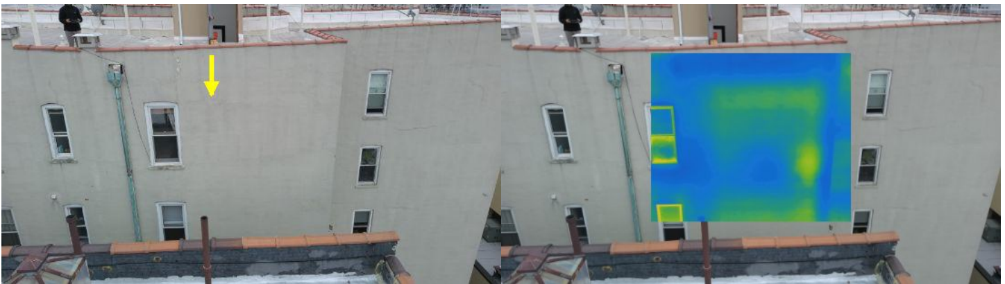
Water entering through side facade and parapet wall coping stone, cascading down and depositing into the wall areas below.
