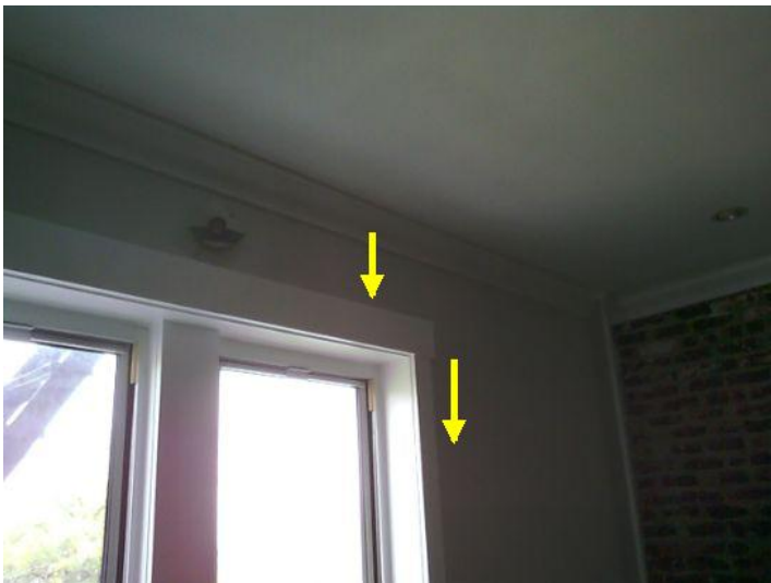
Water entry into wall / window frame area.
