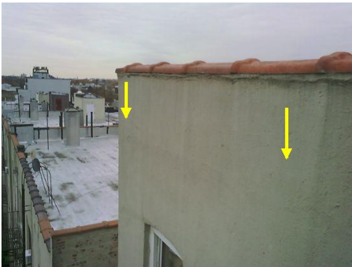
Water entering through the parapet wall coping stone and cascading down into the internal wall areas below.
