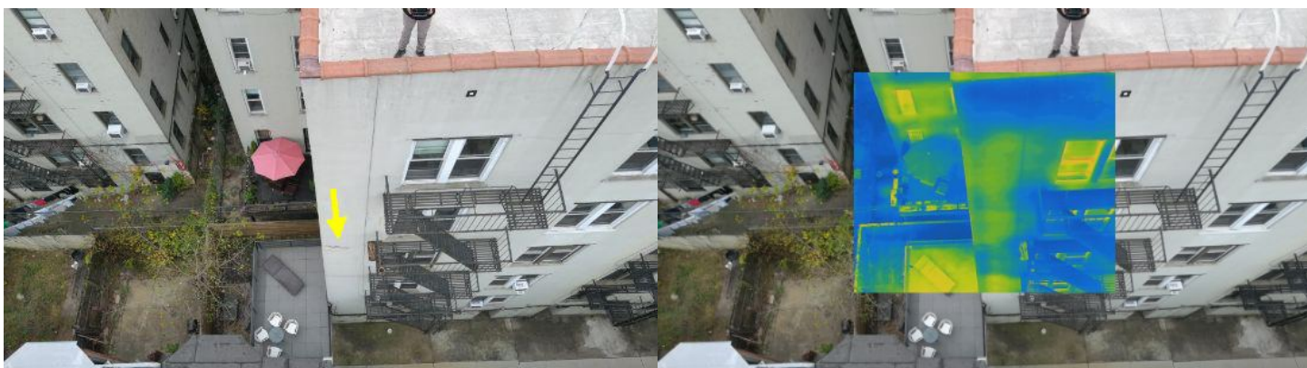
Water entering through the rear facade and parapet wall coping stone, cascading down and depositing into the wall / window frame areas below.
