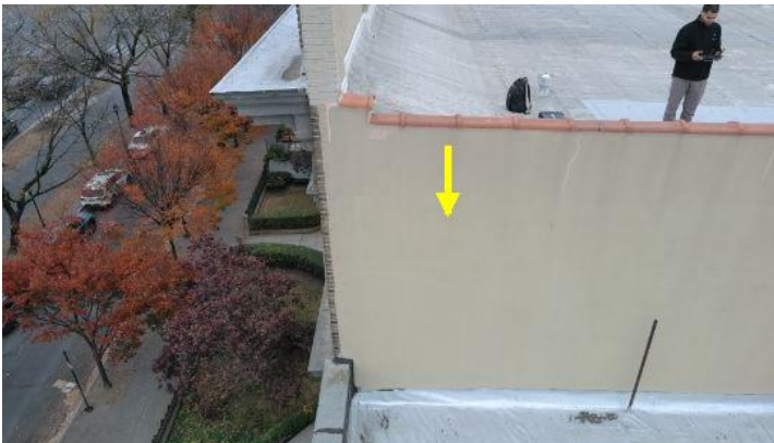
Water entering through the parapet wall coping stones and cascading down into the wall areas below.
