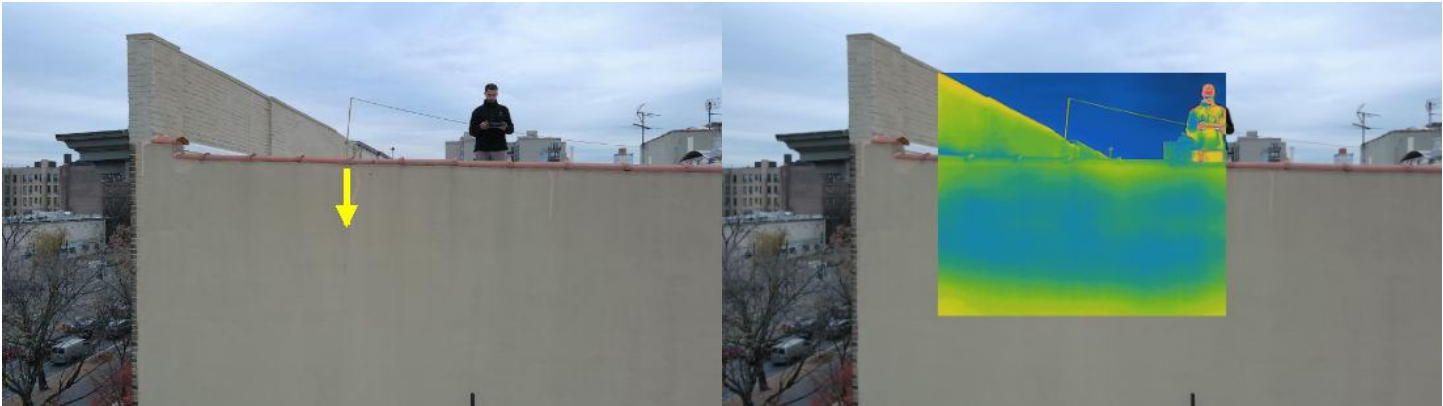
Water entering through the parapet wall coping stones and cascading down into the wall areas below.
