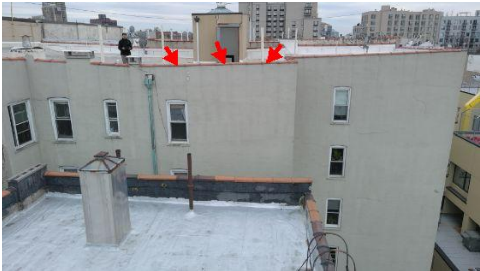
Repair Point: Remove coping stones from parapet wall. Waterproof side facade. Waterproof parapet wall.
