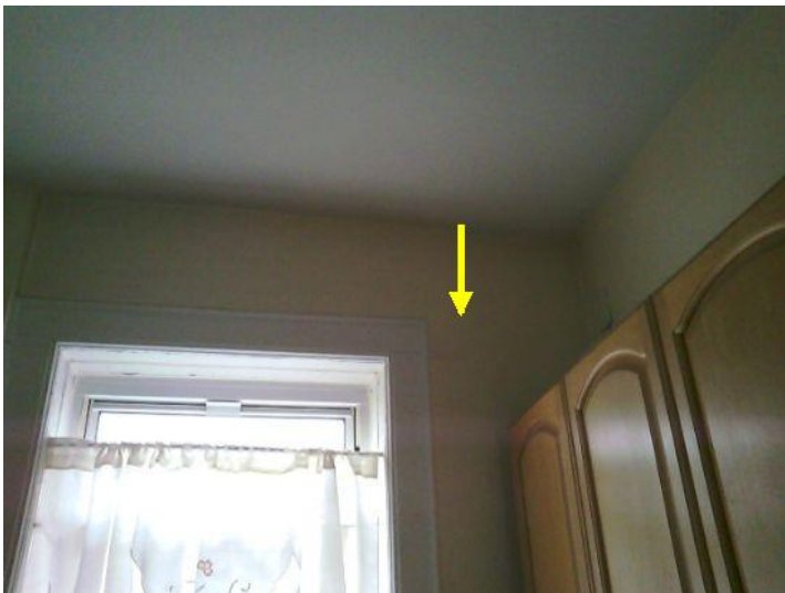
Water entry into wall area.
