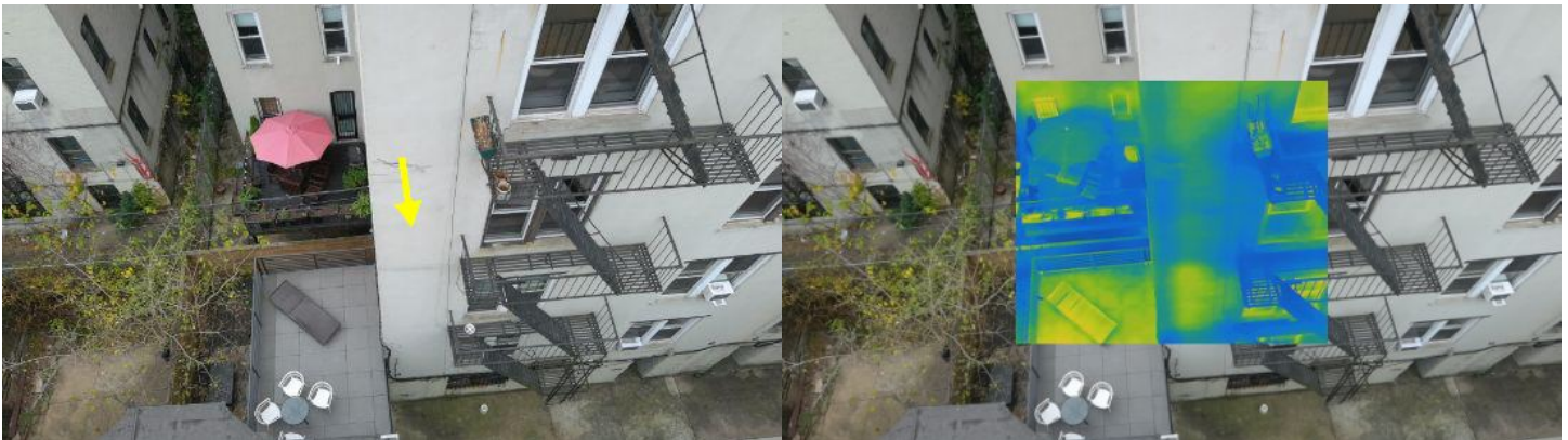
Water entering through the rear facade and parapet wall coping stone, cascading down and depositing into the wall areas below.
