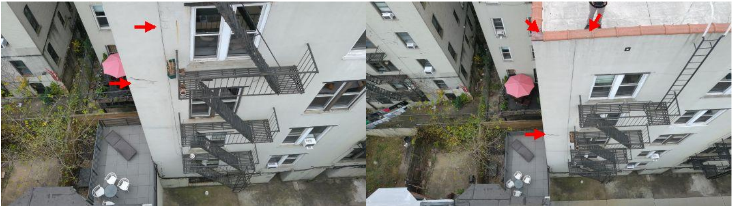
Repair Point: Remove parapet wall coping stones. Waterproof parapet wall. Waterproof rear facade.
