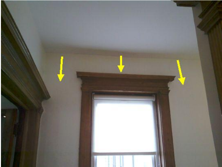
Water entry into wall / window frame area.
