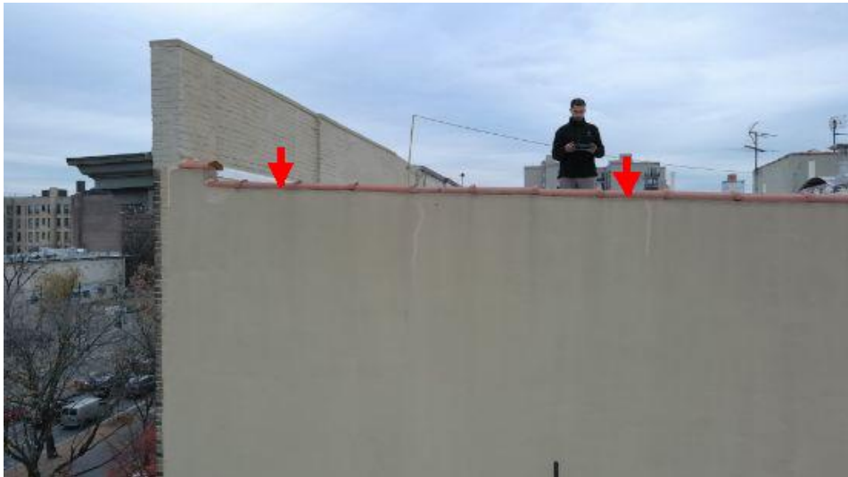
Repair Point: Remove parapet wall coping stones. Waterproof parapet wall.....
