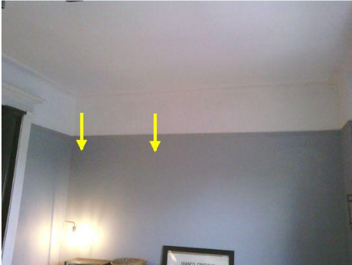
Water entry into wall area.
