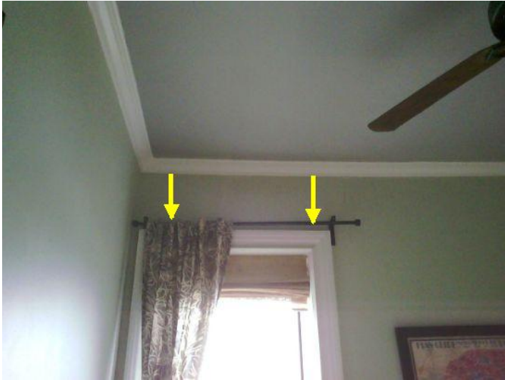
Water entry into wall / window frame area.
