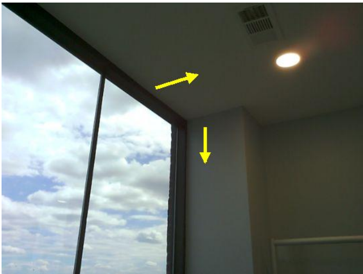
Water entry into window frame area.
