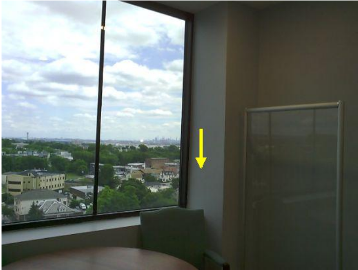
Water entry into window frame area.
