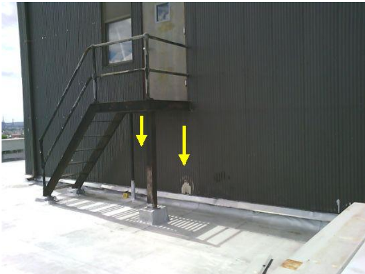
Water entering through the bulkhead wall panels around the door baseplate and window, cascading down and depositing into the ceiling areas below.
