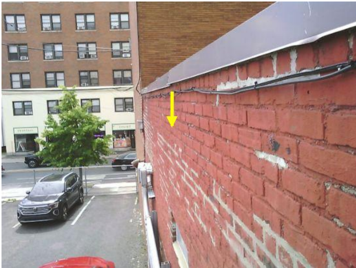
Water entering through parapet wall flashing cap joints and outer brick facade, cascading down and depositing into the wall areas below.
