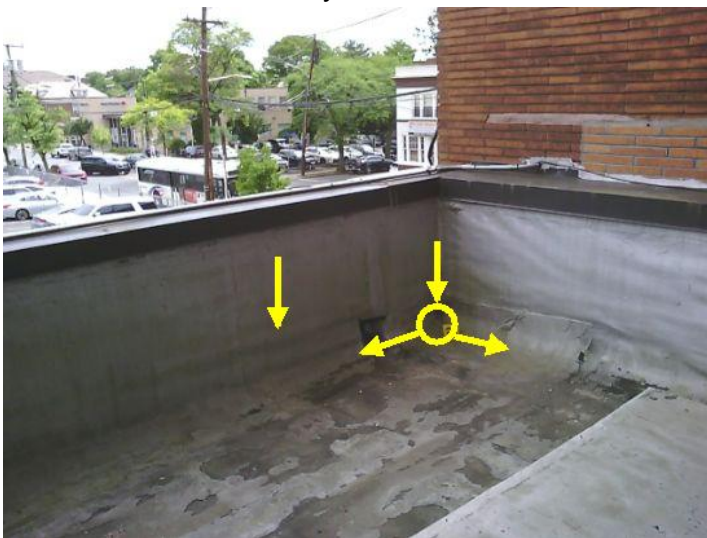
Water entering through the parapet wall flashing cap joints and connecting brick facade, cascading down and depositing into the wall areas below.
