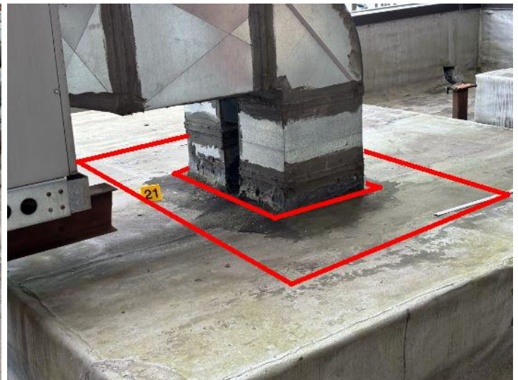
Repair Point: Seal outlined area of roof membrane system with Polyglass 1C liquid roof flashing or similar type material.
