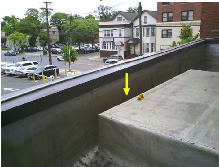
Water entering through parapet wall flashing cap joints and outer brick facade, cascading down and depositing into the wall areas below.
