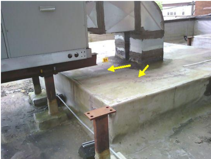
Water entering through HVAC duct entry point into the roof membrane system and cascading down into the wall areas below.
