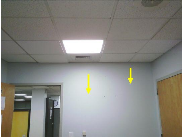
Water entry into wall area.
