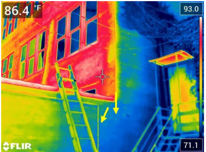
Infrared imaging of water entering through brick facade connection point to the parapet wall and cascading down into the internal ceiling / wall areas below.
