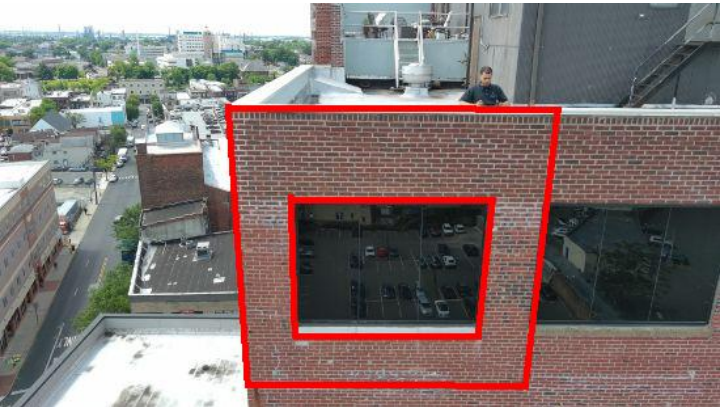
Repair Point: Seal upper facade around window frames with an Elastoflex-type sealant system.
