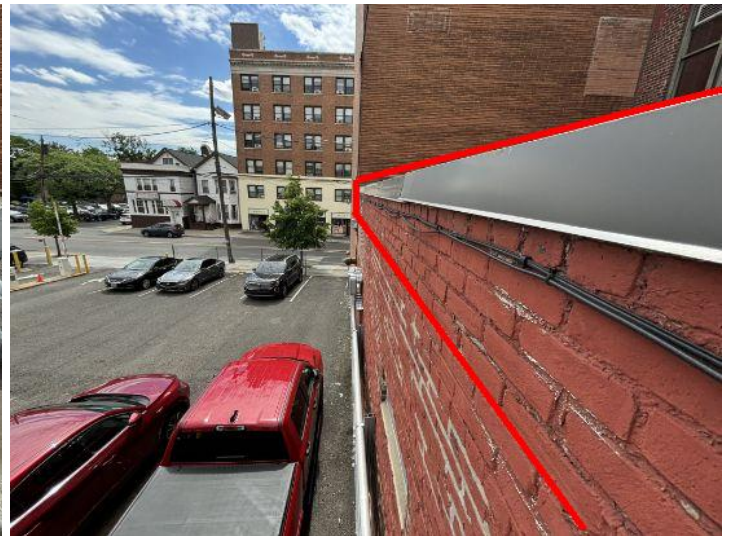
Repair Point: Remove flashing cap from parapet wall. Waterproof rear brick facade. Waterproof parapet. Install new flashing cap.
