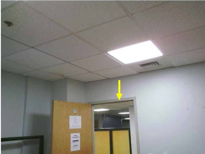
Water entry into wall area.
