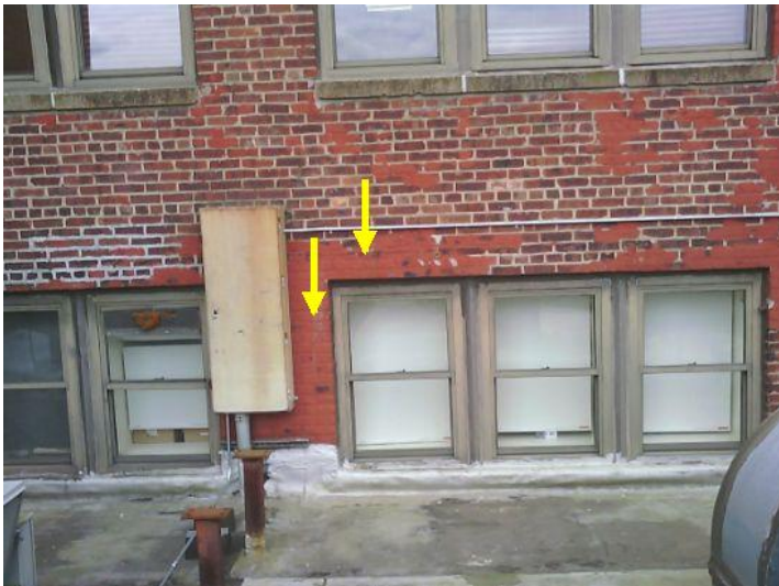
Water entering through the window sill and brick facade areas, cascading down and depositing into the internal wall areas below.
