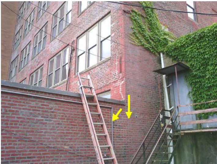
Water entering through brick facade connection point to the parapet wall and cascading down into the internal ceiling / wall areas below.
