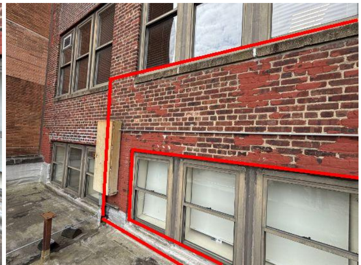
Repair Point: Waterproof window sills and brick facade area. Waterproof deteriorated section of roof membrane with a liquid roof flashing such as Polyglass 1C.
