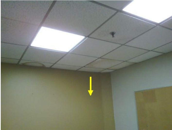
Water entry into wall / ceiling area.
