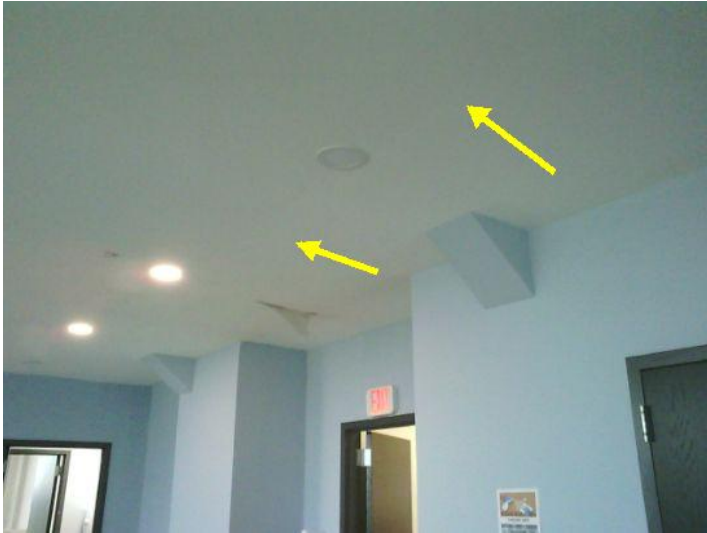
Water entry into ceiling area.
