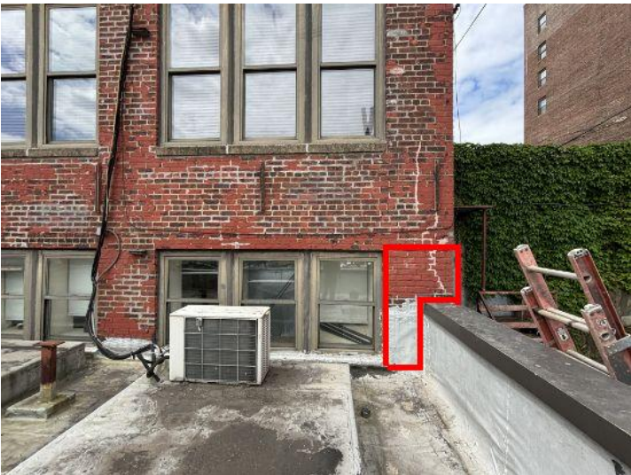
Repair Point: Waterproof brick facade connection point to the parapet wall.
