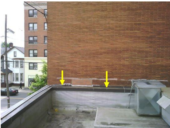
Water entering through the parapet wall flashing cap joints and connecting brick facade, cascading down and depositing into the wall areas below.
