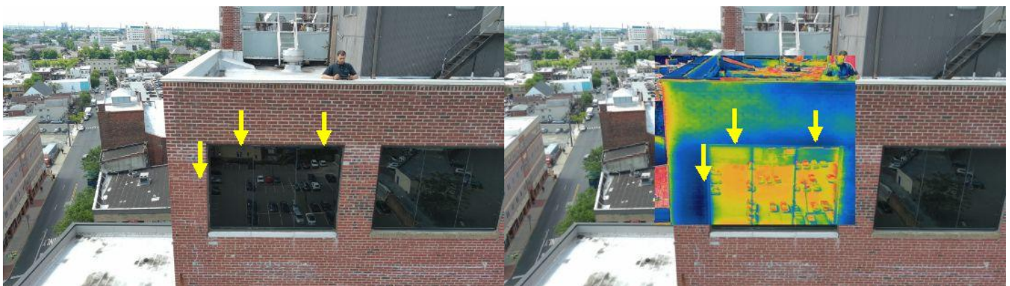
Water entering through the brick facade and cascading down into the window frame areas below.
