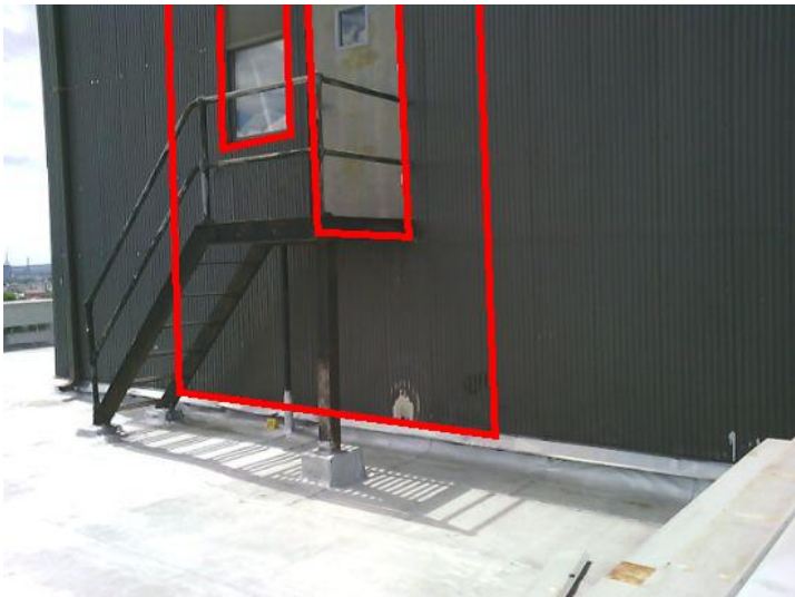
Repair Point: Remove panels from bulkhead wall around window and door frame. Waterproof and flash areas accordingly.
